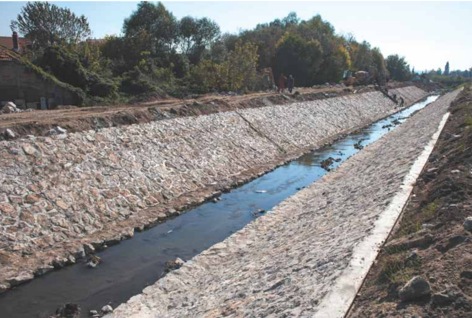
Smederevska Palanka, Regulation and cleaning of the bed of the Ivak stream, cost of works around €162,000
